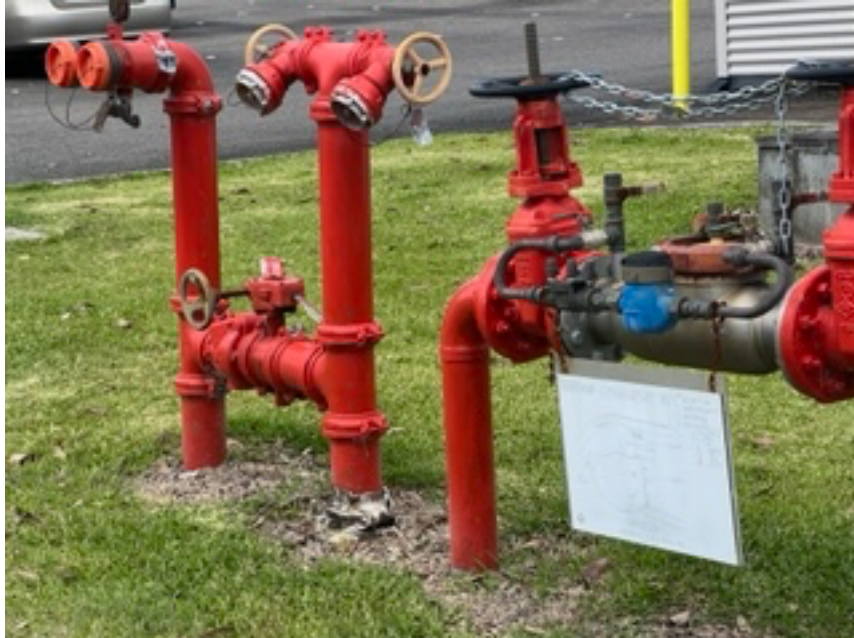
Photo 5. Hydrant Assembly (Source: HVBCS 12/12/2021)
